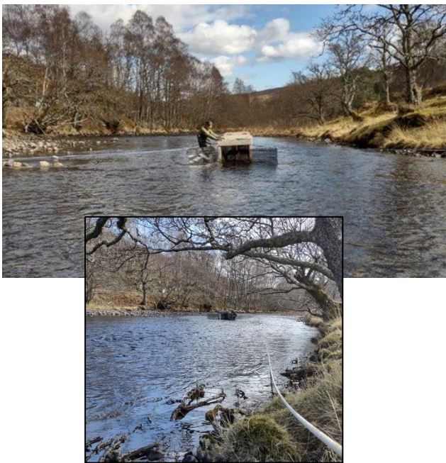
Photo 5: Farrar West Arm box trap (Strathconon), NH 26484 38037. Double wing intercepting flow.
