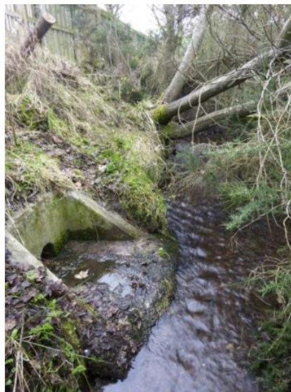
An outfall on Bridgend burn, March 2023
