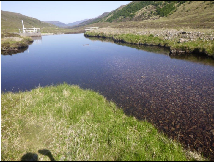
Photo 3: Pile of managed substrate placed out of the active channel, upstream of the Farrar weir. NH22102 38915
