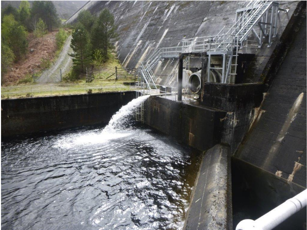
The base of Mullardoch dam with compensation flow, Glen Cannich
